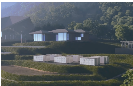
REMOTE AREA OFF-GRID
